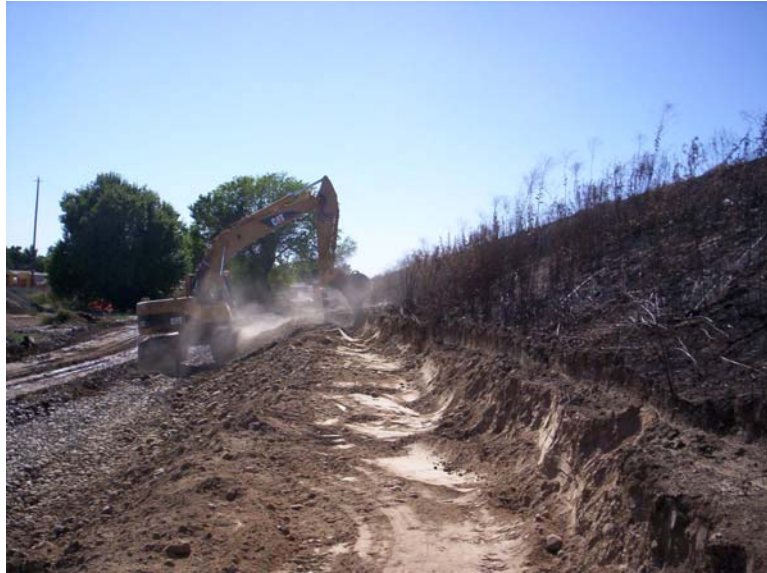
Photo 2: Yuba Seepage Berm – Cobble Removal and Benching
