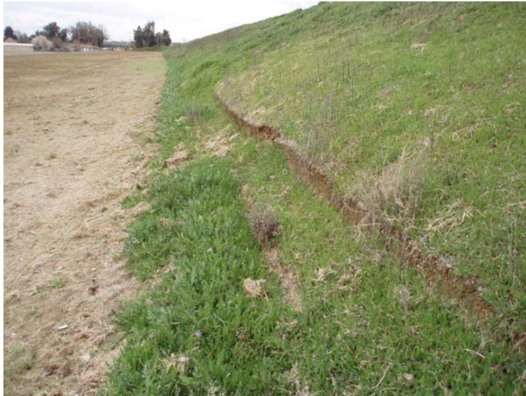
Photo 4: Yuba River Levee Scrape January 2007
