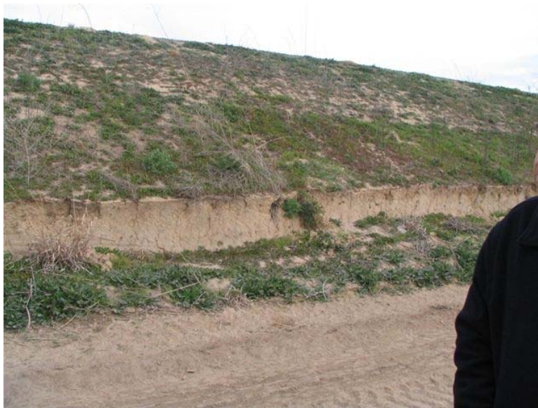
Photo 5: Yuba River Levee Scrape February 2007
