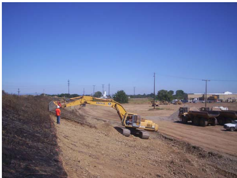
Photo 1: Yuba Seepage Berm - Cobble Removal
