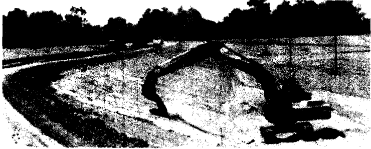
Construction of Bear River Levee
